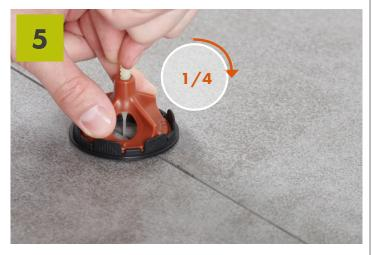
7. Now go back to the first installed SOS Rescue Clip and tension it by turning the cap by another quarter turn; keep a firm hold of the upper handle.
