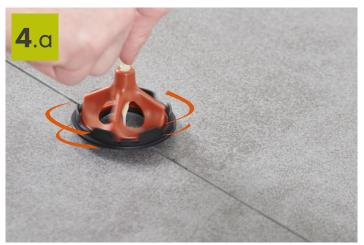
5. Tension the clip by tightening the cap by <u>one quarter</u> <u>turn.</u>
