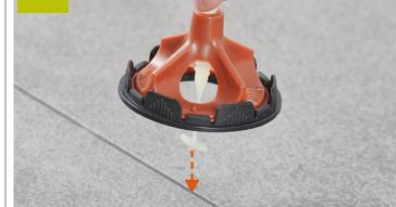
3. Holding the upper handle with your fingers, rotate the SOS Rescue Clip by 90° (until the grip is perpendicular to the joint).
