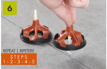
8. Now go back to the second installed SOS Rescue Clip and tension it by turning the cap by another quarter turn; keep a firm hold of the upper handle.
